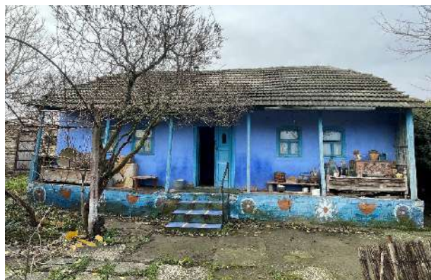
Image 3. Façade of the renovated old house, v. Oxentea. Photo: Ivanova Nina, 02.12.2024
