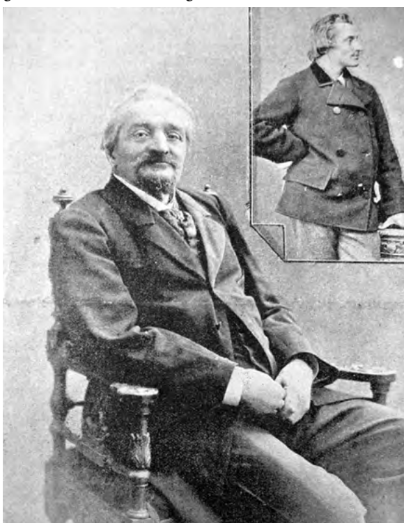
Architect A. Bernardazzi (1831–1907)
