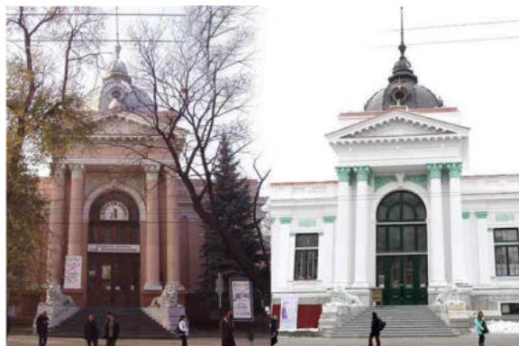
Fig. 5. Kishinev Organ hall before and after restoration.
