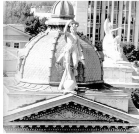
Fig. 4. Sculptures adorning the building of Kishinev city public bank.
